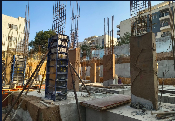
Column Reinforcement
